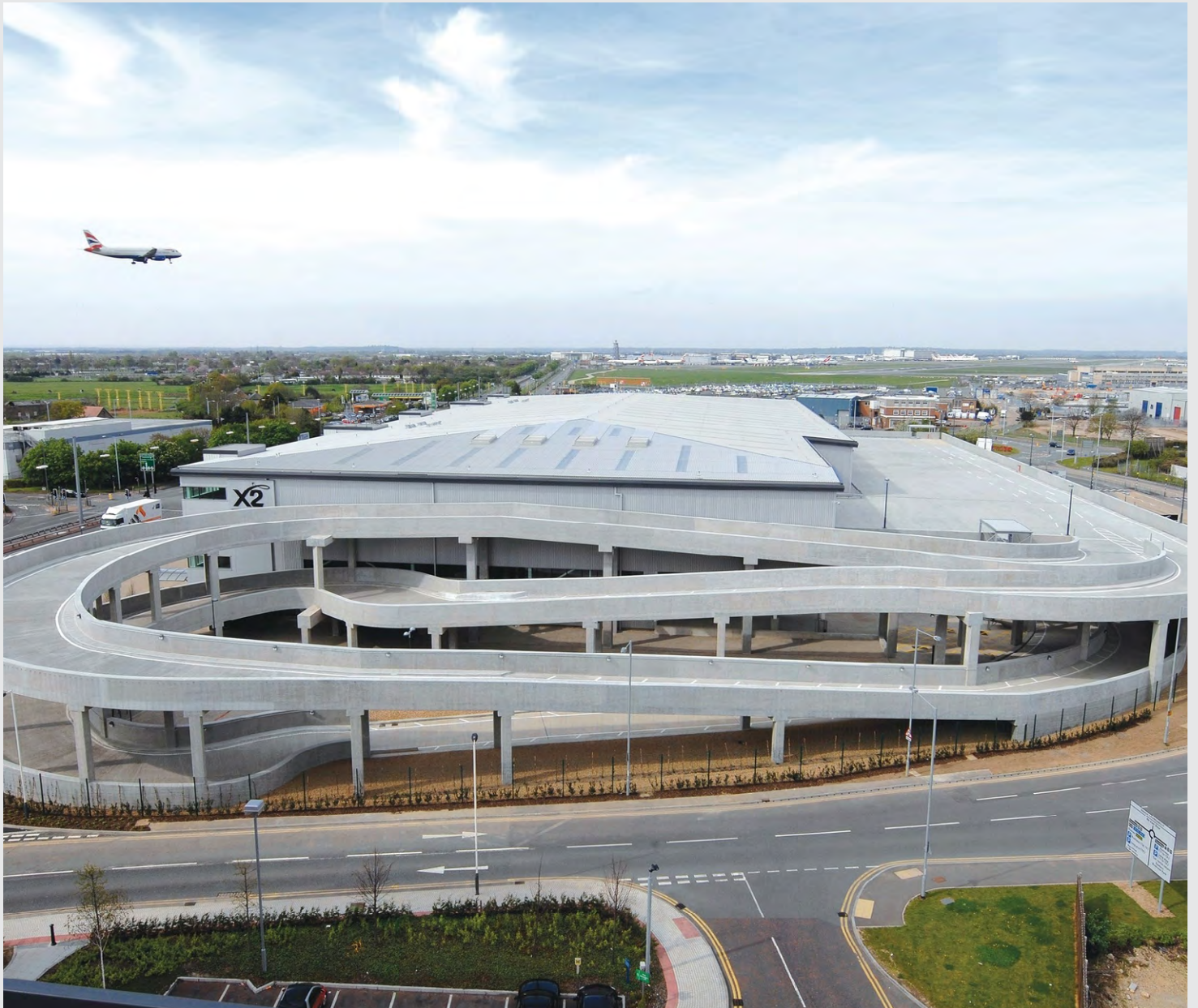
X2 warehouse, Hatton Cross - Multistorey warehousing with access ramp. Cornish Architects
