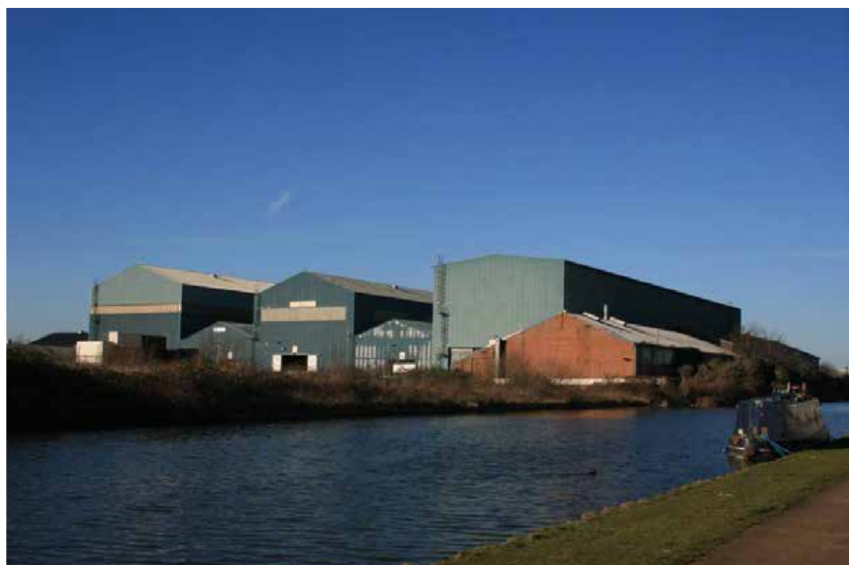
Warehouse 5 and 6 (right) on the Meridian Water site
